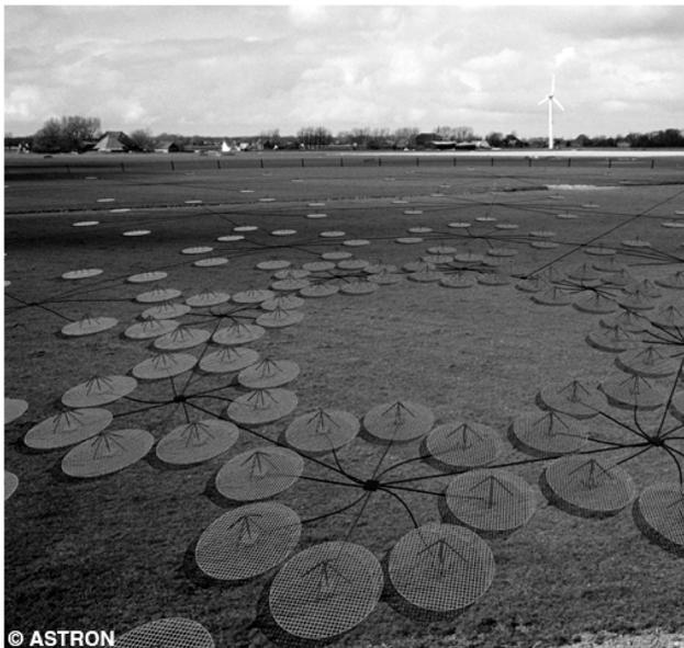
**Figure 5:** Model of a LOFAR station with low-frequency antennas (by courtesy of ASTRON).
